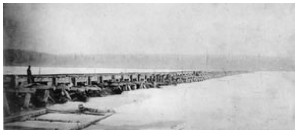
The Rice Lake Bridge showing the trestles used
