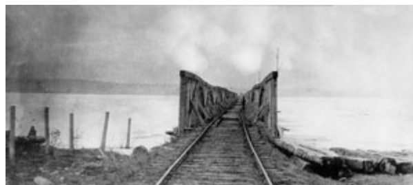
Rice Lake Bridge - probably taken after being damaged.
